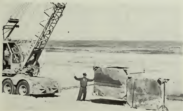
LOTS OF PULL —Cat skinner pulls pontoons from bay with dozer ( rt ) and crane lines up sea wall on eroded beach.
